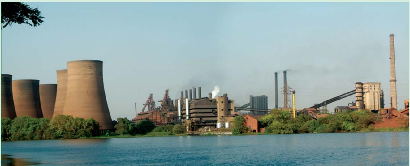
A panoramic view of SAIL's IISCO Steel Plant.
