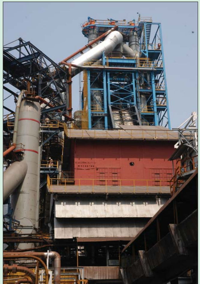
View of a Blast Furnace.
