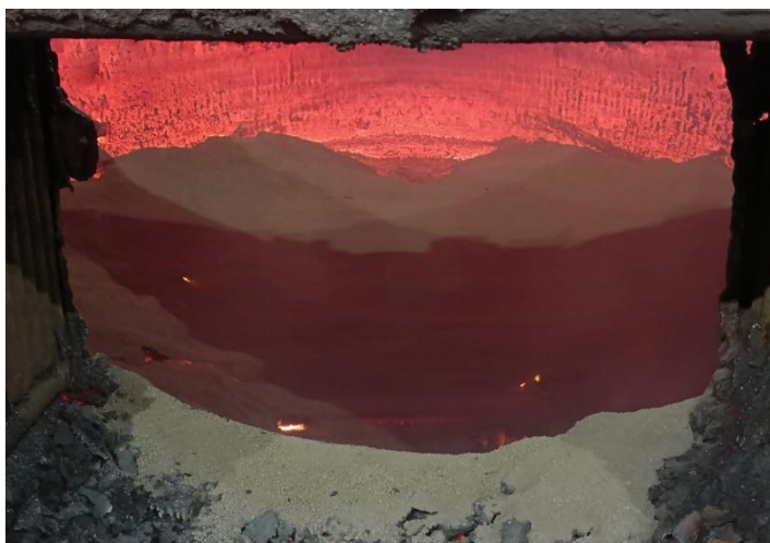
Hot repair with Dry ramming mass
