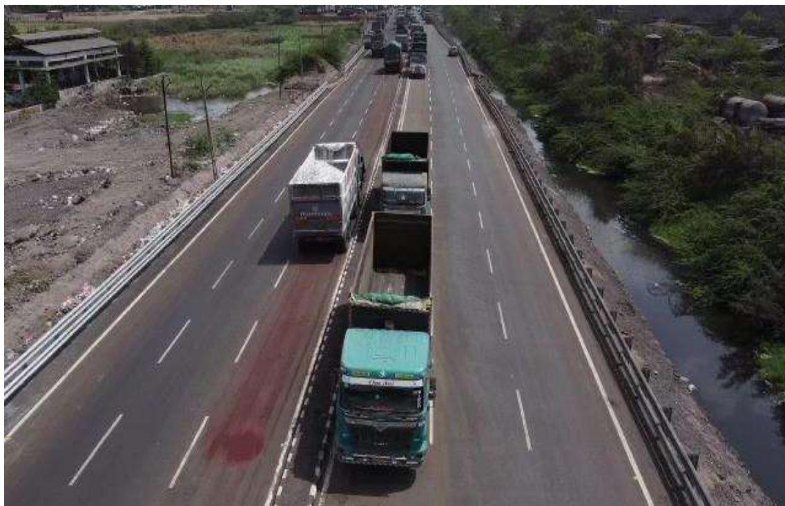
Photo A.1: Aerial view of Six Lane Bituminous Steel Slag Road built at Hazira Surat using processed EAF Steel Slag Aggregates
