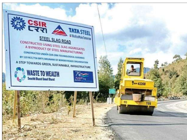
Photo A.5: Glimpse of Steel Slag Road Section Built at Ziro, Arunachal Pradesh by BRO
