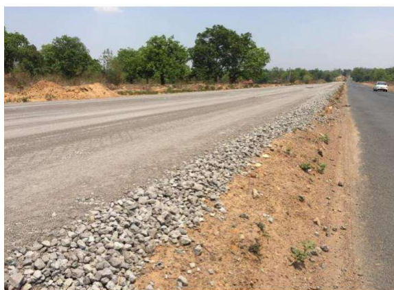
Photo A.6: BOF Steel Slag Aggregates in GSB and WMM layers of NH 33 on natural soil embankment
