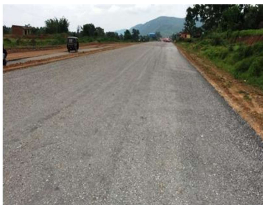
Photo A.7: WMM layers with steel slag aggregates on NH-33 after prime coat
