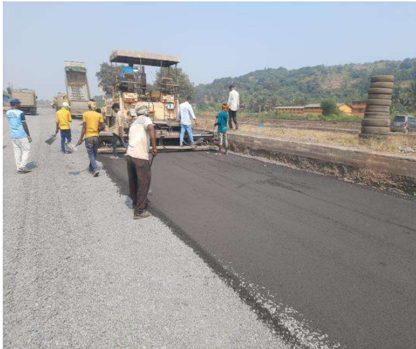
Photo A.3: Laying of DLC layer and Inauguration of NH- 66 (Mumbai-Goa National Highway) steel slag road section by Hon. Member Niti Aayog Dr. V.K.Saraswat
