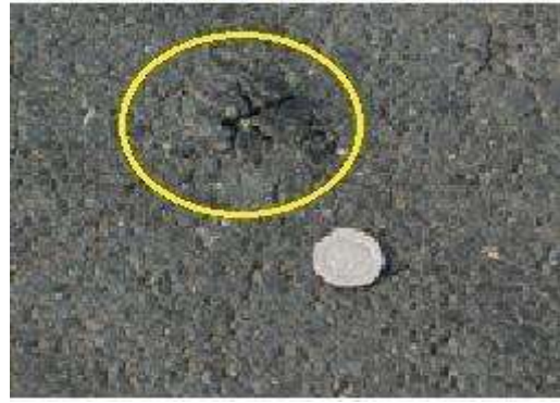
Photo 3.2: Heave in bituminous layer due to Volumetric expansion in slag aggregates
